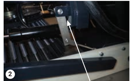
2-3 mm gap between the metal and the A-frame
